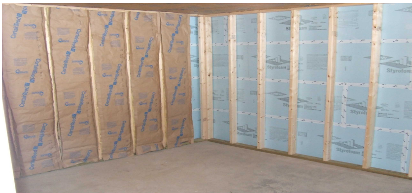
example of 15/19 utilizing R-5 continuous insulation
