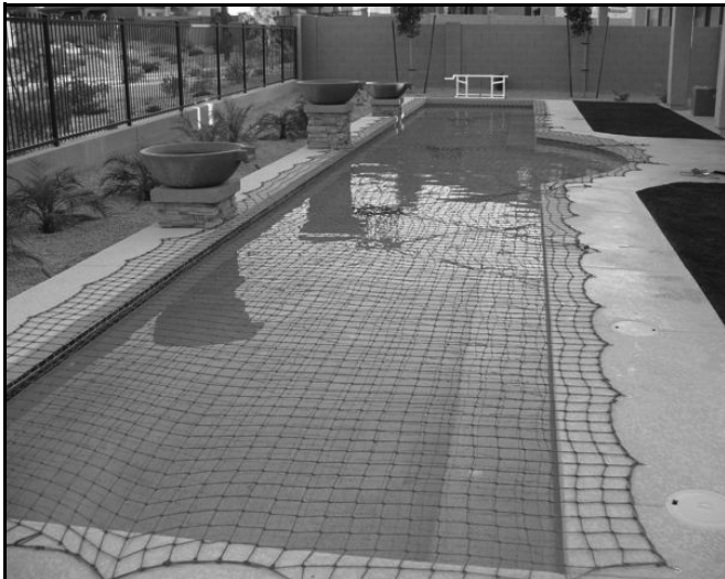
FIGURE 305.1(4) NONPOWERED MESH COVER DOES NOT ALLOW FOR ABSENCE OF BARRIER AROUND POOL
