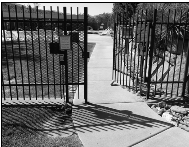
FIGURE 305.3 VIOLATION—WRONG SWING DIRECTION ON PEDESTRIAN ACCESS GATE
