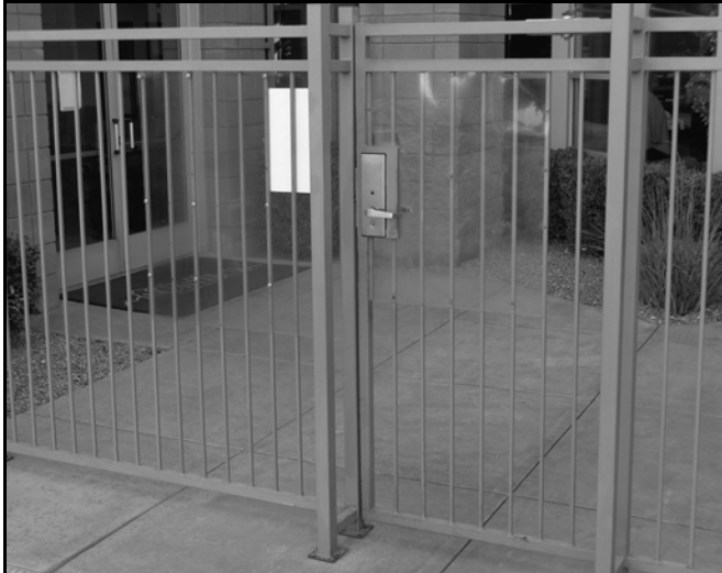
FIGURE 305.2.6(2) VIOLATION—BARRIER (FENCE) HORIZONTAL MEMBERS TOO CLOSE
