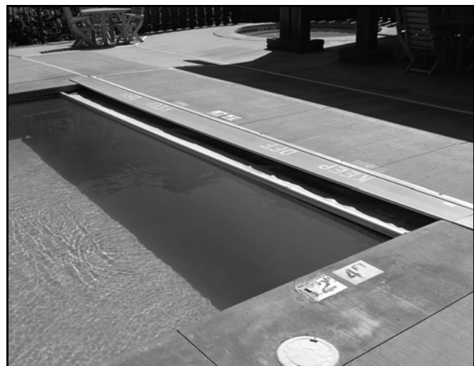
FIGURE 305.1(2) INTEGRAL-TYPE POWERED SAFETY COVER FOR PUBLIC POOL
