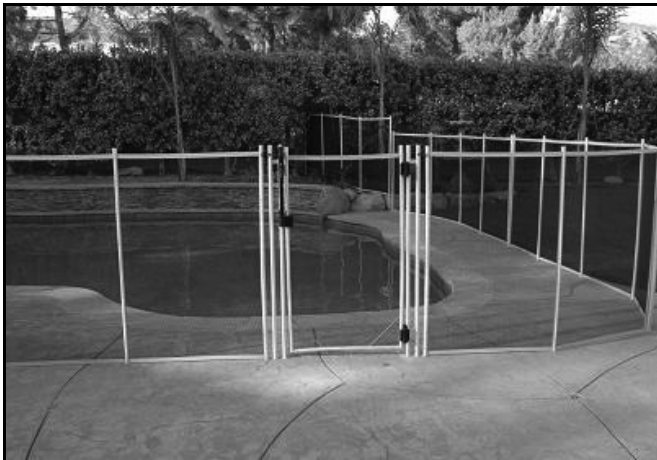
FIGURE 305.2.4 MESH FENCE AS A STRUCTURE- TO-POOL BARRIER
