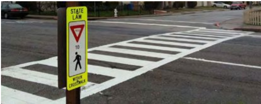
Figure 4: Ladder Style Crosswalk
