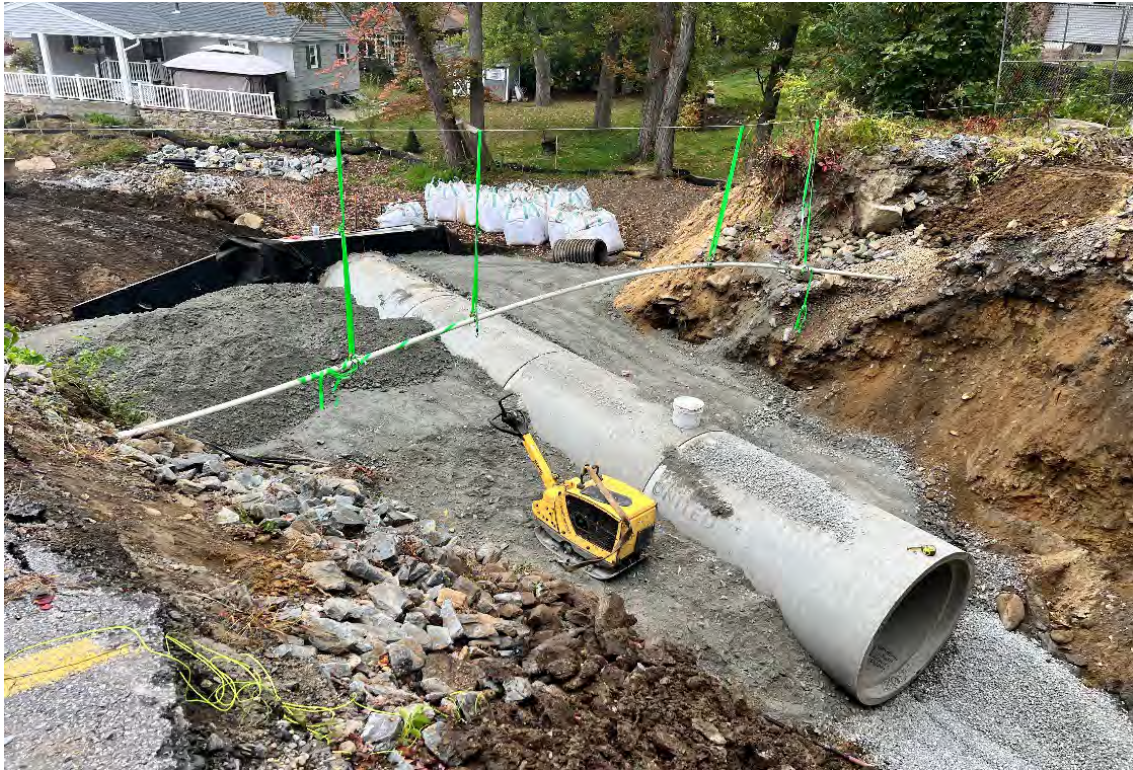
Pictured above is the 48-in drainage pipe which now conducts stormwater to the Assabet River.
