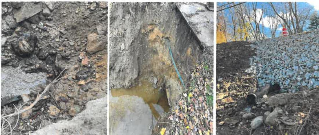
The 100-year old culvert at Brigham Street has collapsed. Temporary pipes have been installed to allow water to flow at about 40%. A fully-designed and constructed replacement is needed to replace this culvert.
