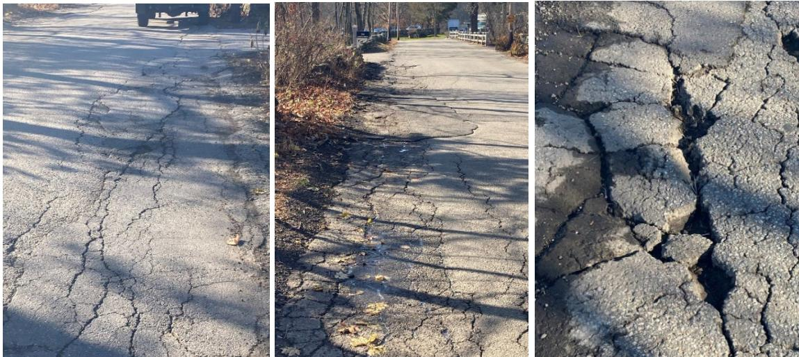
The current poor condition of Lewis Street, with extensive spalling, has been caused by the absence of a stormwater collection system. The road has been damaged by routine flooding.
