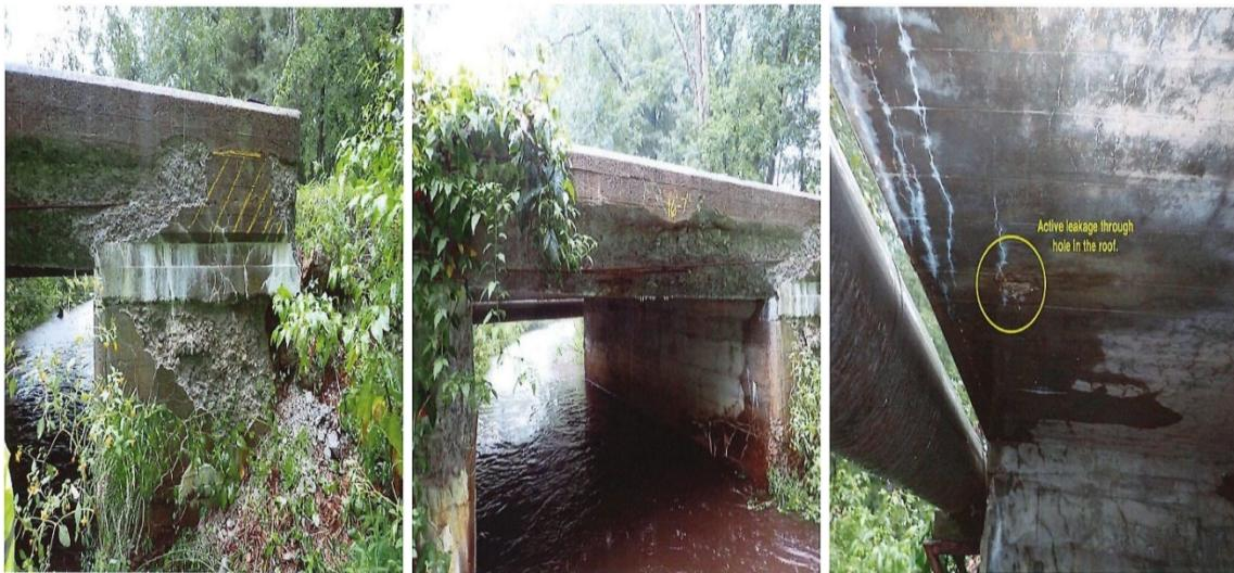
The culvert and bridge at Shay Road have significant deficiencies and are in need of full replacement in the not-too-distant future.
