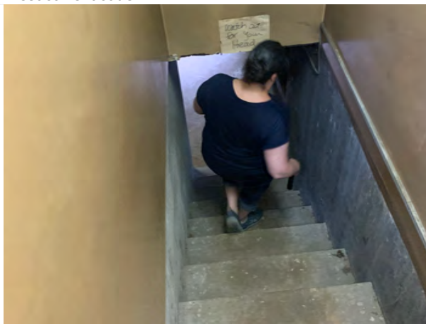
The staircase to the boiler room in the basement has no code-required handrails; and has insufficient headroom, which is a code violation and a safety hazard for technicians and Town personnel.
