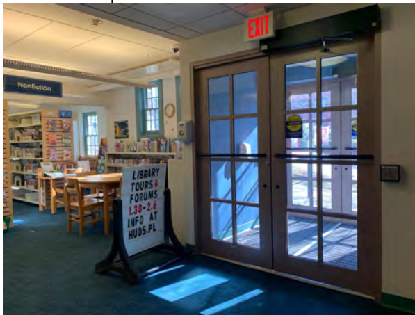
Aluminum doors with push-button handicap-accessible hardware were installed at the Children's Room south side entrance in 2001.
