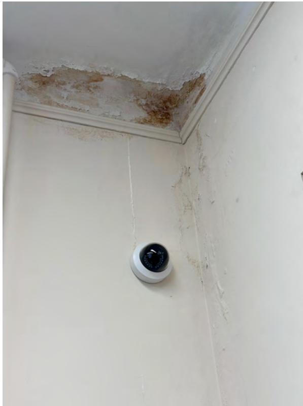
The brick walls of the southeast corner of the Carnegie Building's 1 st Floor (teen space) have a persistent leak, causing peeling plaster at the interior.
