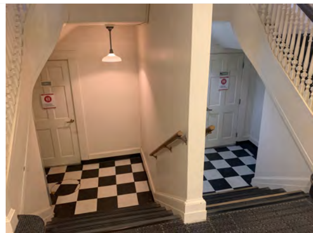
Historic stairs to the bathrooms below the Ground Floor do not have compliant handrails.
