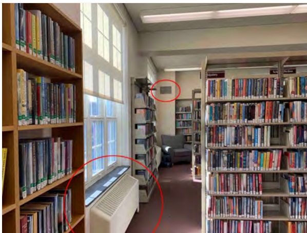
Heat is delivered through steam radiators below the windows of the 1st Floor 1966 Addition; air conditioning is delivered through grilles in the two rear corners of the room.
