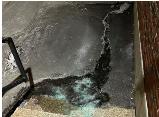
Slip hazard due to unplumbed downspout at staff entrance exterior stairs bottom landing.
