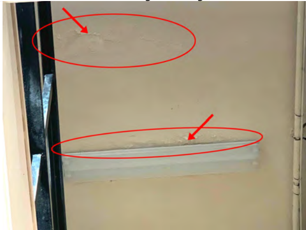
Peeling paint on the ceiling of the north exit stair tower is evidence of current roof leaks.
