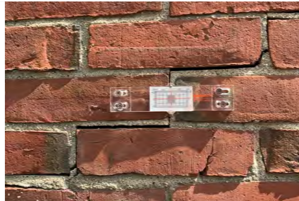
Mortar is in poor condition due to cracking at the facades of the 1966 Addition.
