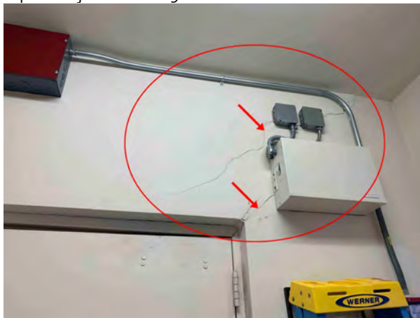
Cracking wall at the staff kitchen door leading to the boiler room, at the rear of the Ground Floor. Cracking indicates uneven settlement of brick wall and foundations.
