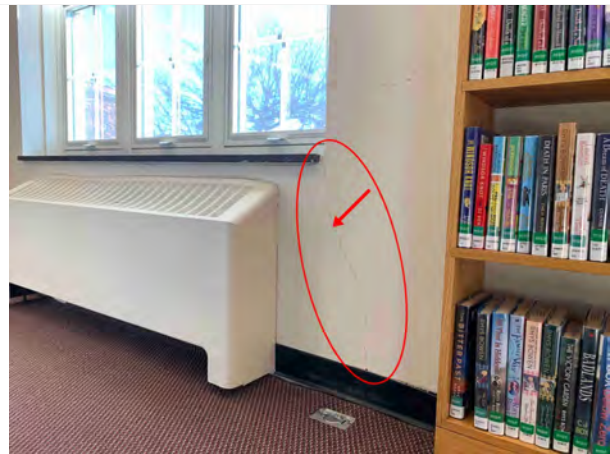
Cracking sheetrock wall at the rear of the 1st Floor. Cracking indicates uneven settlement of brick wall and foundations.
