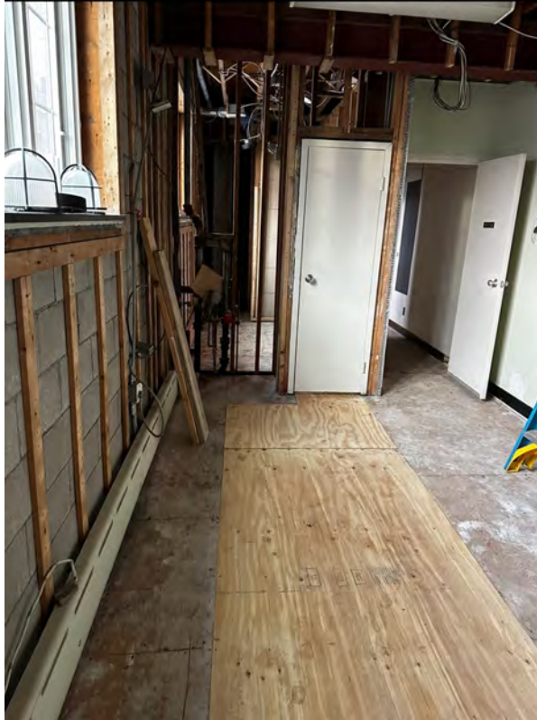
Extensive plumbing pipe replacement occurred for sinks and toilets during repair from the April 2023 steam pipe leaks. This was due to condensation filling wall and ceiling cavities and causing corrosion on plumbing piping.
