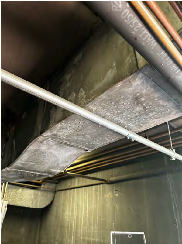
Condensation observed on July 20, 2023 on the surface of the unjacketed Zone 3 ductwork in the boiler room.
