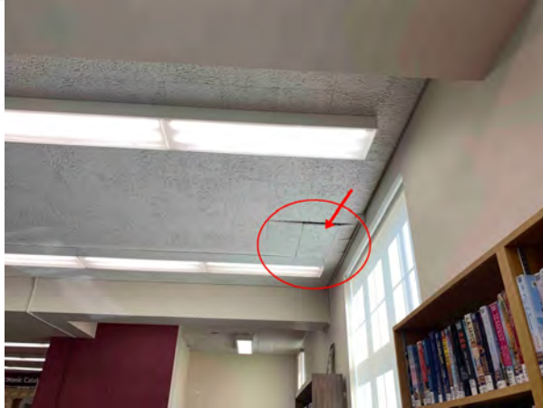
Evidence of roof leak in the ceiling of the 1st Floor, 1966 Addition.
