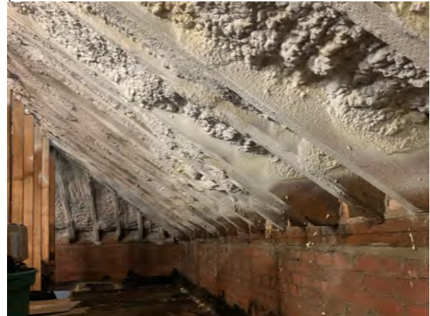
Four inches of spray foam were added to the underside of the Carnegie Building roof in 2022.
