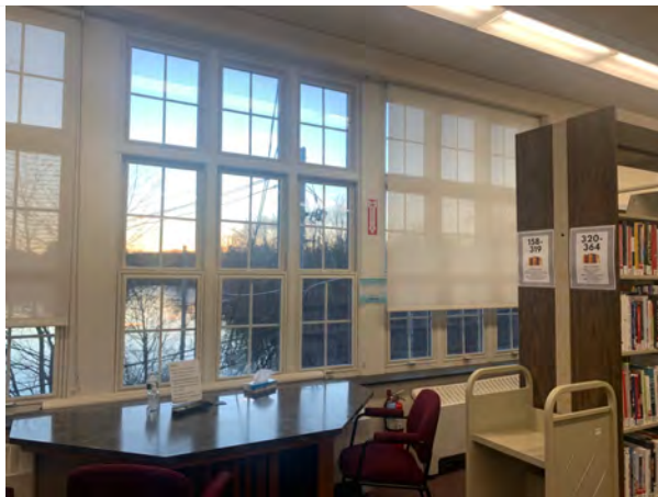
Typical interior view of a 2010-installed aluminum replacement window in the 1966 Addition.
