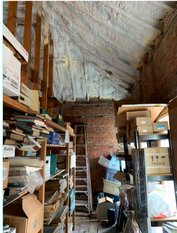
Combustible materials higher than 8 ft and combustible spray foam insulation on the inside of Attic roof.
