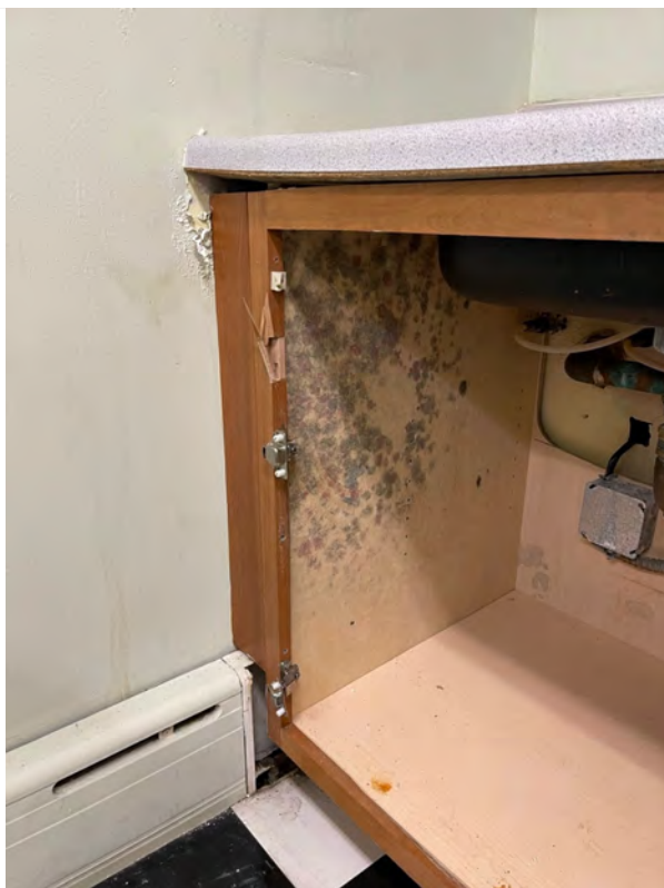
Mold was found on surfaces in the staff kitchen and restroom due to steam pipe leaks.
