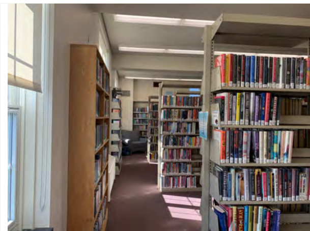
Metal shelving on the 1st Floor violates building code due to the weight of its contents; the floor diaphragm was designed for a "Reading Room" not a "Collections Room."
