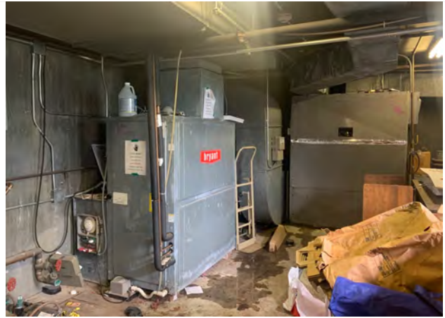
The 10-ton AC air handler for the 1966 Addition portion of the 1st Floor is located in the boiler room.
