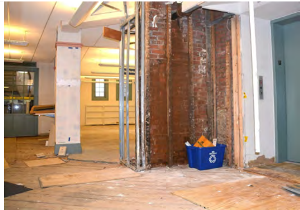
Repairs to Children's Room after steam pipe leak at Ground Floor elevator soffit, Spring 2021. Photo credit Ed Karvoski Jr., Community Advocate
