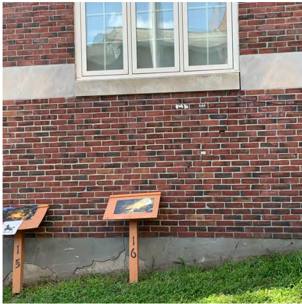
Cracks along 1966 addition side facing Liberty Park.
