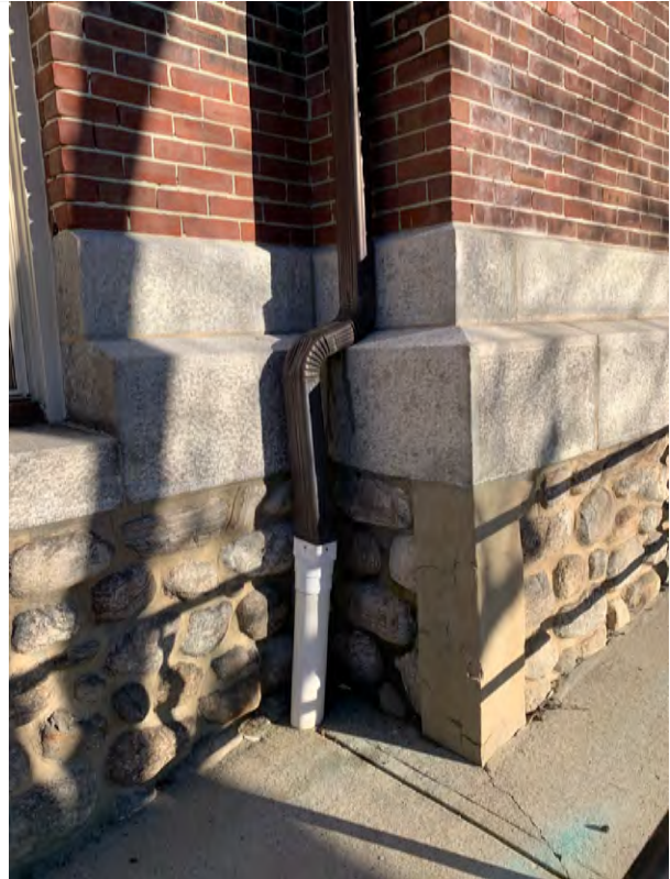
Some downspouts are correctly plumbed to storm piping such as this downspout on the south side of the building.
