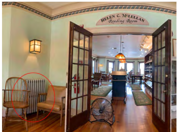
Heat is delivered through hot water radiators throughout the 1st and 2nd Floors of the Carnegie Building.
