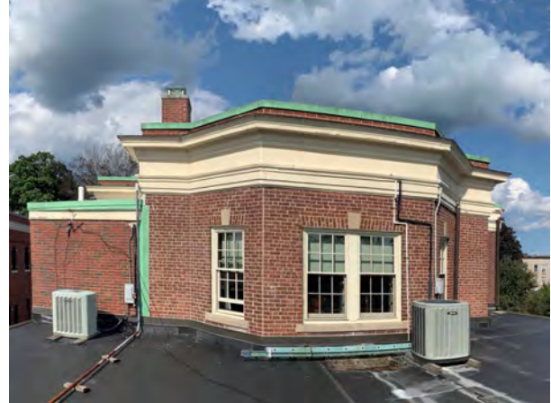
The roof of the Carnegie Building is a patina green-colored PVC membrane installed in 2010; deco-ribs added to the pitched areas make it look like a metal roof.
