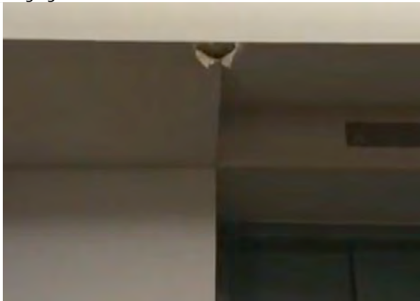
Steam pipe leak at Ground Floor elevator soffit, Spring 2021.
