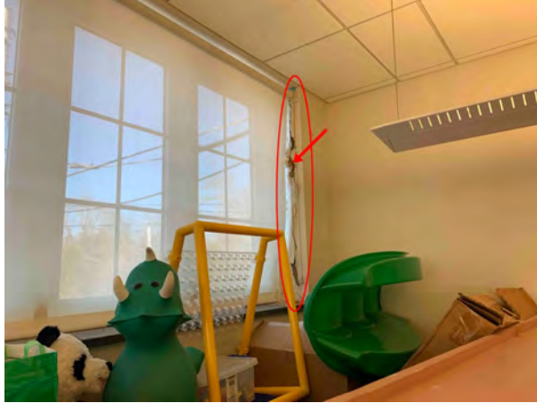
Active leak at Children's room Ground Floor rear window.
