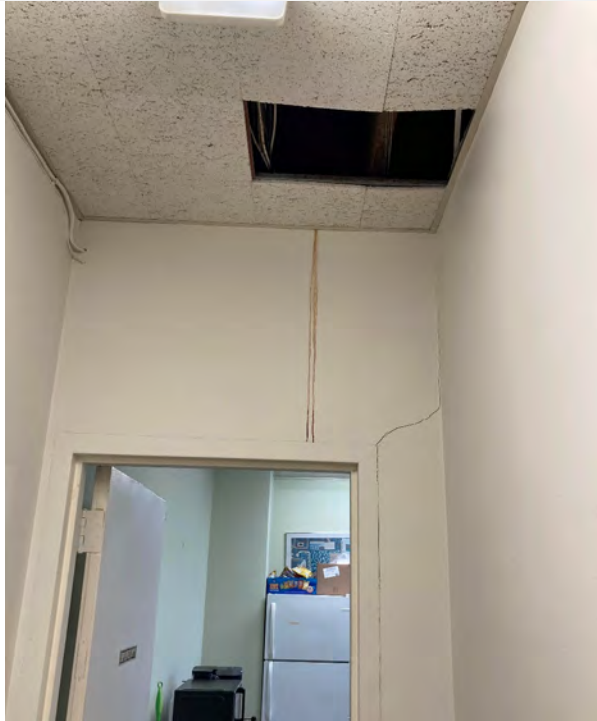
Steam pipe leaks at the Ground Floor concrete floor chase, resulting in steam buildup, mold and mildew in the staff area ceiling in April 2023.
