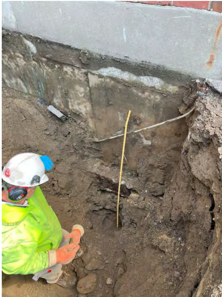
Test Pit TP-2 Excavation, Looking East. Note exposed bottom of footing bearing within the fill layer.
