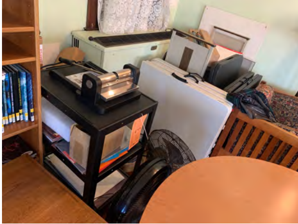
A UniVent forced air heater serves the McLellan Room. However this unit works intermittently and should be replaced.
