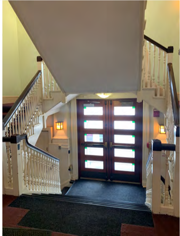
Historic stairs at the front of the Carnegie Building have non-code-compliant guardrails and handrails.
