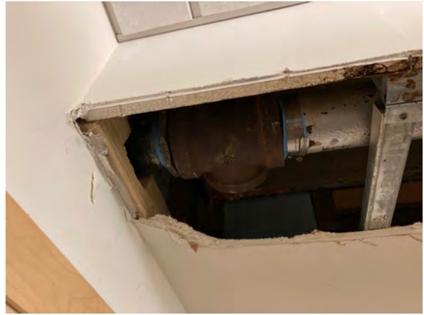
Steam pipe leak at Ground Floor elevator soffit, February 2024.
