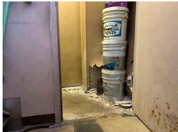
The exterior wall at the boiler room top stair landing is crumbling due to uneven settlement and water intrusion. The boiler room door (foreground) is rusted.
