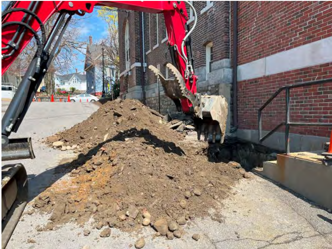
Test Pit TP-2 Excavation, Looking Northeast. Note the quantity of cobbles and boulders within the uncontrolled fill.
