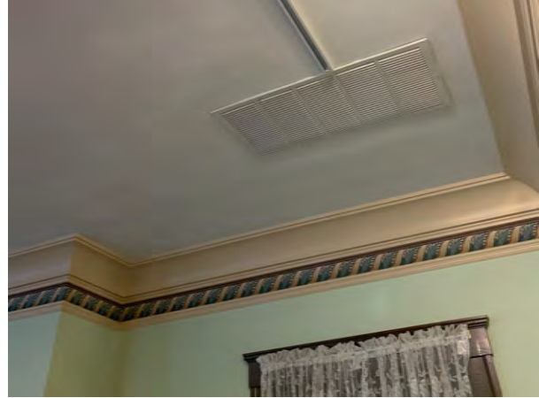
Air conditioning registers are located on the ceiling of the McLellan Room, directly below an AC unit. Too much cold air is delivered via the registers, and excess AC is directed to the circulation desk area below by conventional fans.
