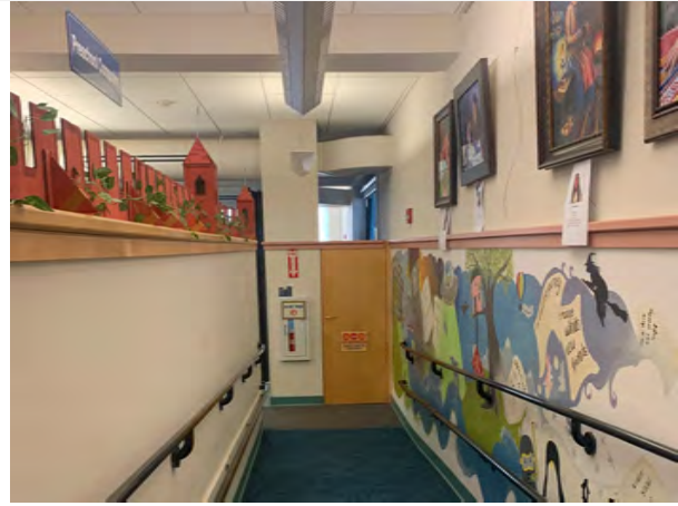
The craft room is accessed via this non-code-compliant door at the bottom landing of the ramp in the Children's Room.
