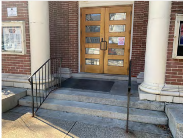
Main entry stairs and handrails are not handicap-accessible. Landings at the front doors are not code-compliant.
