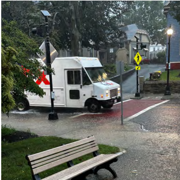
Water ponds at the crosswalk in front of the Library during storm events, causing an icy puddle, a potential slip hazard, in winter.
