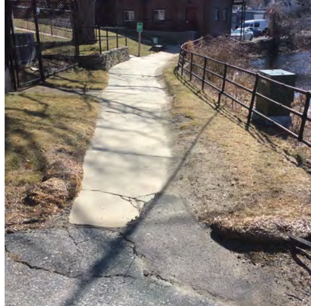
View from north of the cracked and uneven sidewalk used to access the Library from the adjacent public parking lot.
