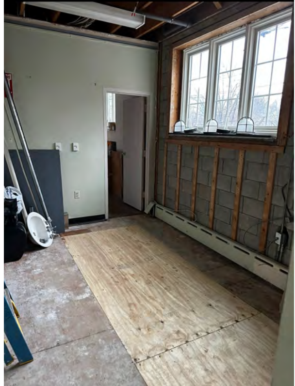
The contractor who replaced the cabinets in the staff kitchen due to the April 2023 steam pipe leaks found that the floor slopes 2 inches over 15 feet (due to uneven settlement of the building foundation).
