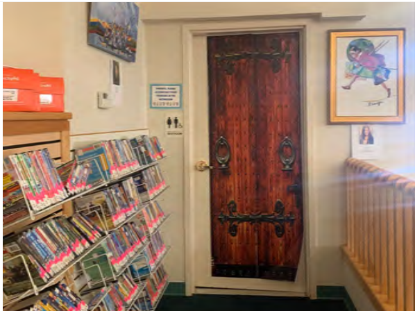
Handicap-accessible restroom does not have sufficient push-side clearance at the entrance to the room and is therefore not code compliant.
