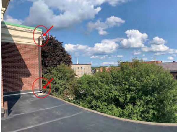
Downspouts from the Carnegie Building roof are not correctly plumbed to drain onto the roof of the 1966 Addition without overflowing or leaking.
