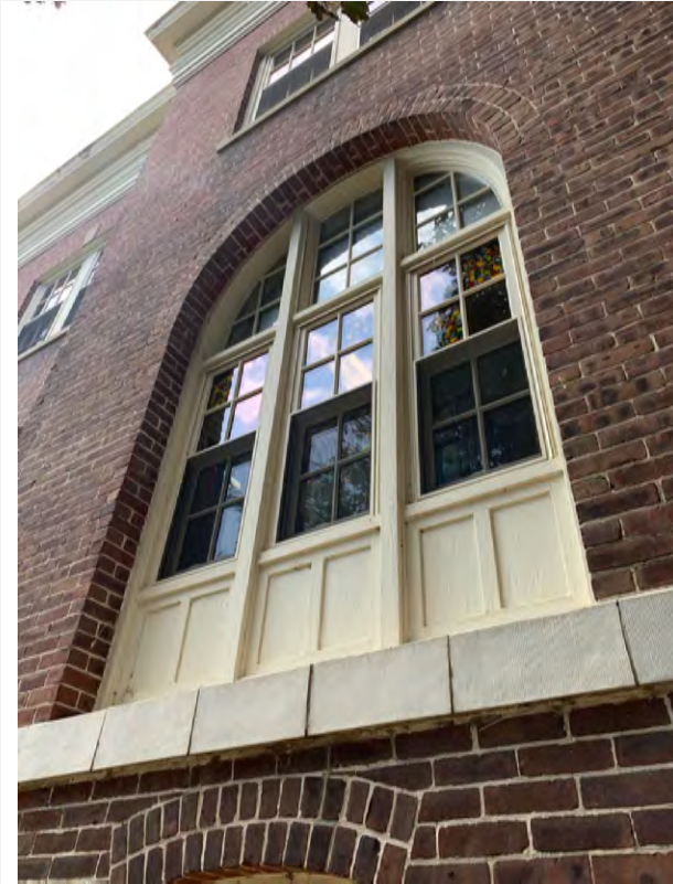
Replacement windows installed in 2010 in the Carnegie Building include painted wood panels, a maintenance concern, rather than durable factory-coated aluminum.
