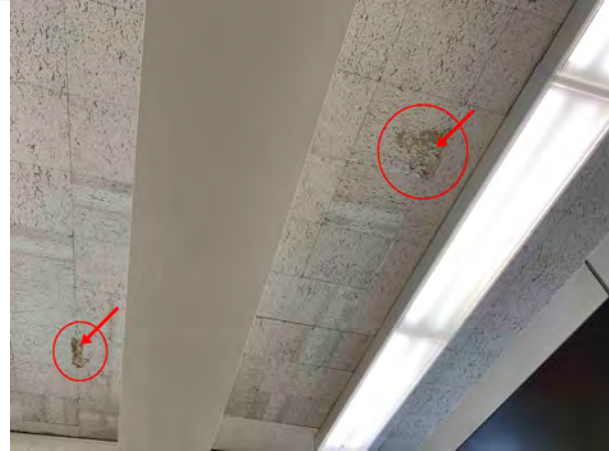
Evidence of roof leaks in the ceiling of the 1st Floor, 1966 Addition.
