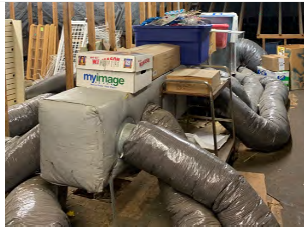
The AC air handler for the 2nd Floor is located in the attic of the Carnegie Building.
