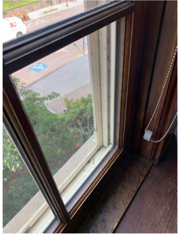
Windows in the Carnegie Building installed in 2010 are wood-wrapped divided-lite replacement windows with insulated glazing units (IGUs) with chain-operated shades.
