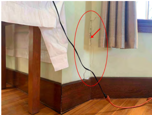
Cracking plaster indicates uneven settlement at the expansion joint for the 1966 Addition.
