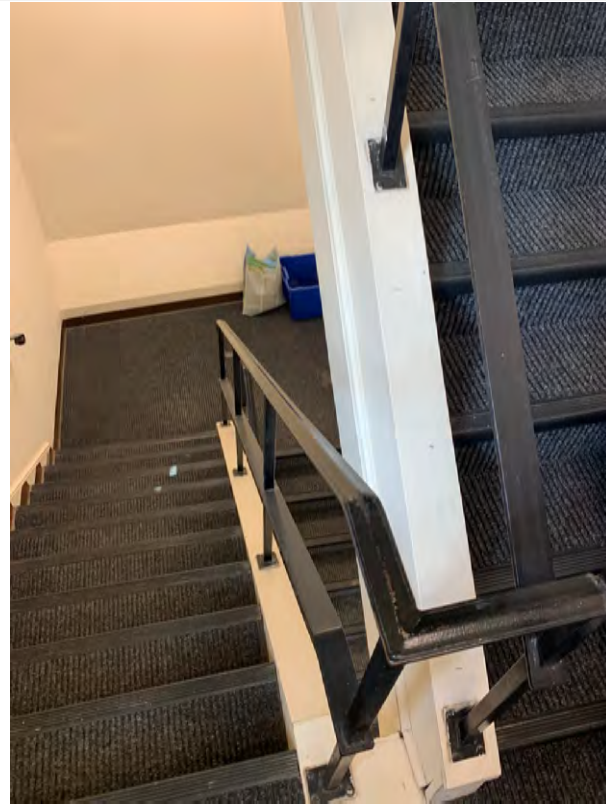
Handrails and guardrails in the egress stair tower do not meet current code.
