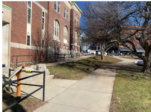
Uphill view of the non-code-compliant ramp on the south side of the building.
