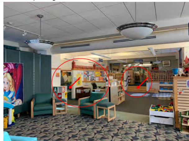
The Children's Room has an unnecessary flight of stairs that resulted in a need to add a ramp to provide handicap accessibility. The change in level is a historic condition based on the space's prior use as a civic meeting room.
