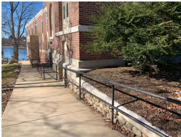
Ramp on the south side of the building designed as the handicap-accessible path of travel has too steep a slope to comply with code.
