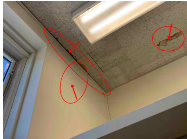
Evidence of roof leaks in the ceiling of the 1st Floor, 1966 Addition; these leaks have also affected the top of the wall, causing bubbling of the sheetrock.
