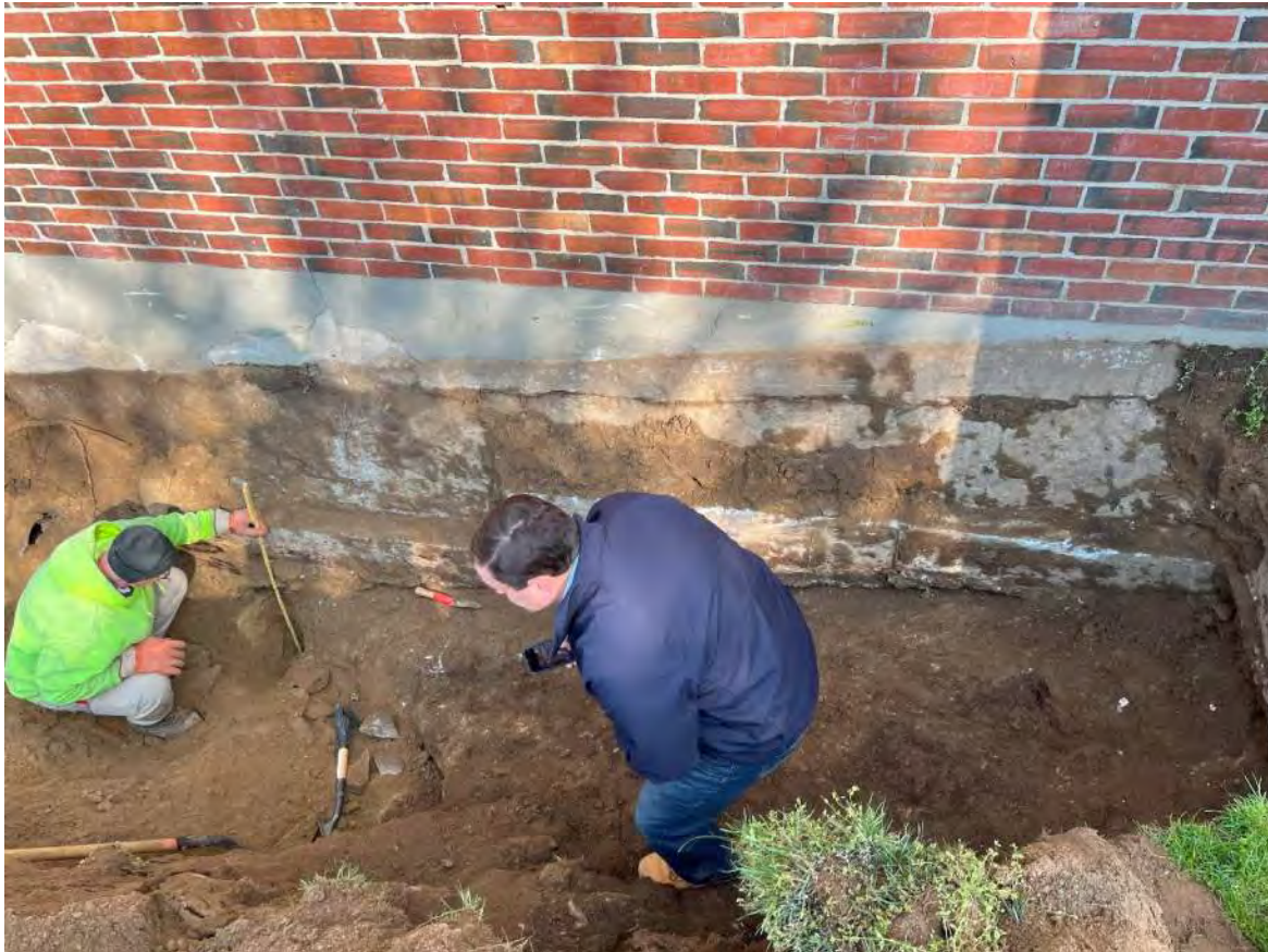
Test Pit TP-1 Excavation, Looking West. Note the edge of exposed bedrock.
