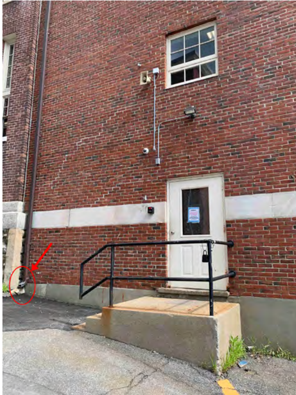
Staff entrance. Image shows downspout is not plumbed to subsurface drainage, leading to a slip hazard due to ponding water at stair bottom landing.
