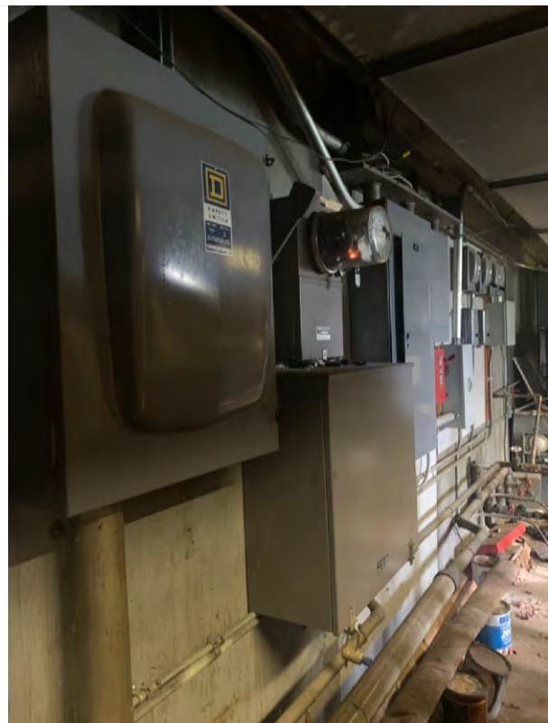
Boiler room electrical panels and disconnect switch.
