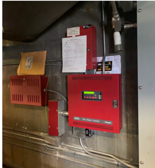
Simplex Fire Alarm control panel is located in the boiler room in the basement, below the 1966 Addition.
