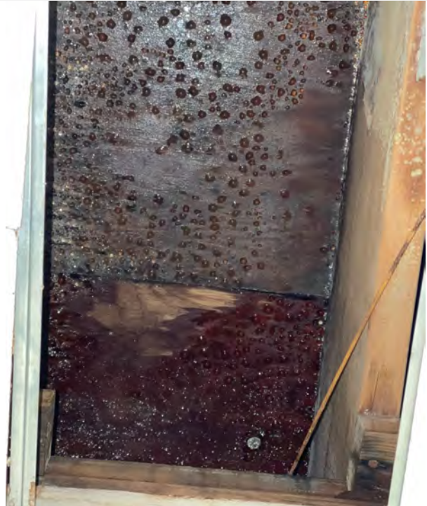
Steam pipe leaks at the Ground Floor staff area in April 2023 – resulting in showing condensation on plywood subfloor of staff area ceiling.
