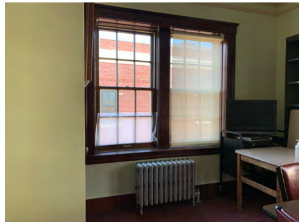
Typical interior view of a 2010-installed wood-wrapped replacement window in the Carnegie Building.
