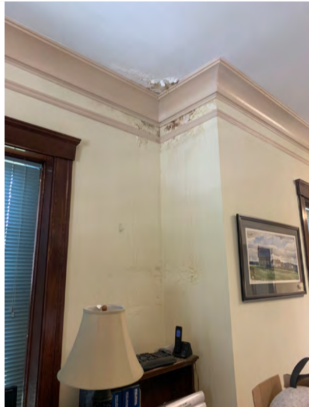
The brick walls of the southeast corner of the Carnegie Building's 2 nd Floor (technical services offices) have a persistent leak, causing peeling plaster at the interior.
