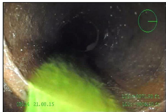
Photo 2 Positive Dye Test during CCTV Inspection
